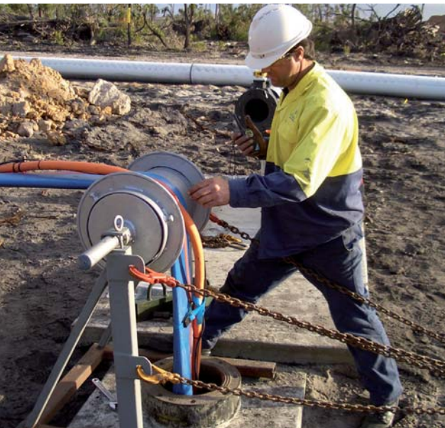
Gently Lower Pump into Bore
