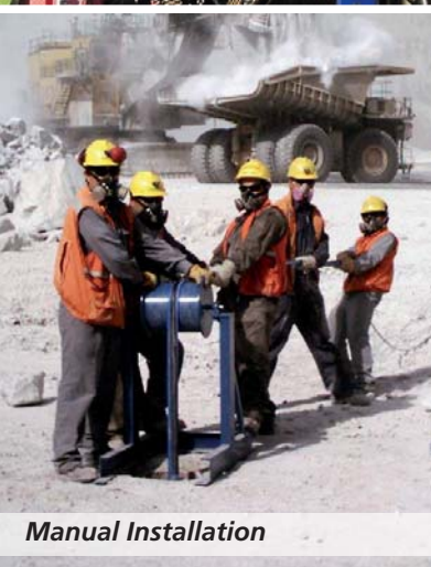
Reel to Lower Pump into Bore
