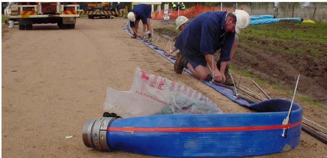
"Snake" power cable to allow for elongation to compensate for the weight of the pump and water etc.
