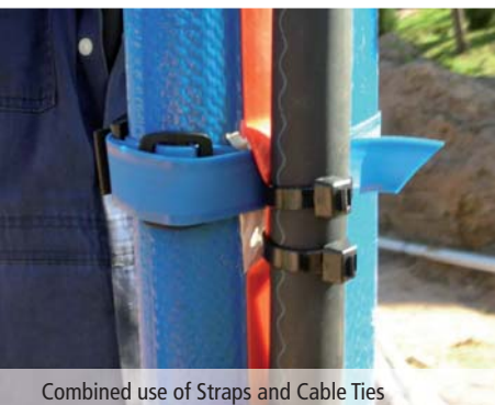
Combined use of Straps and Cable Ties
